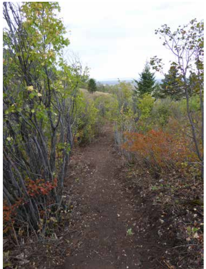
A completed section of trail on September 19 th . The trail’s appearance will improve significantly as understory plants fill-in and native re-seeding takes place, which is scheduled for November 2015.
