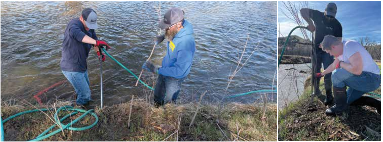
In April, SCLT staff planted willow cuttings at priority sections of Big Goose Creek. It is part of a larger, long-term stream restoration project to stabilize banks, reduce erosion and flood impacts, and improve habitat and access.
